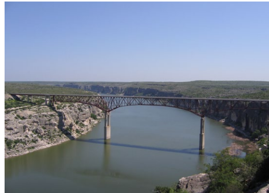
Looking north at the Pecos River Bridge and the Devils River Limestone along U.S. Highway 90.
