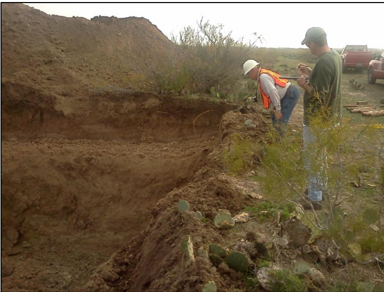
Figure 7 - Site Test Pit
